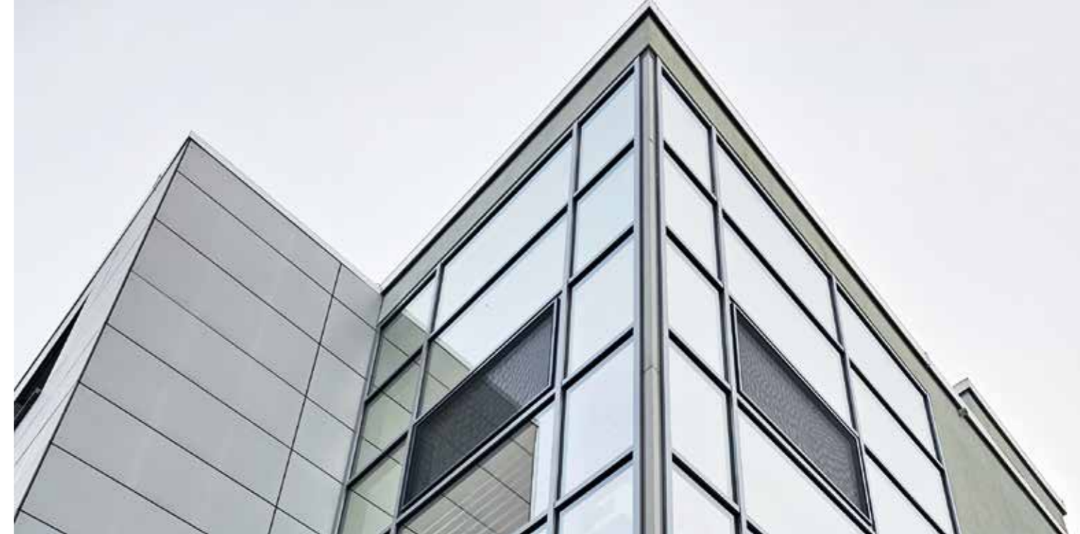
Facade area of the main building of the Fraunhofer WKI in Braunschweig.
